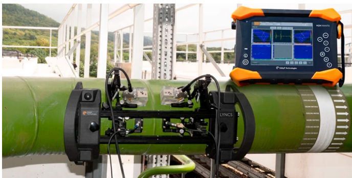
Figure 1: Weld inspection of pipework utilizing LYNCS and Mantis.
